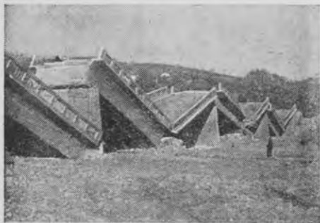
A mined bridge in the forward area.
