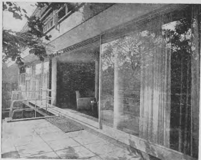
The house in Frognal, Hamstead, showing the large living-room window from the terrace at first-floor level.
