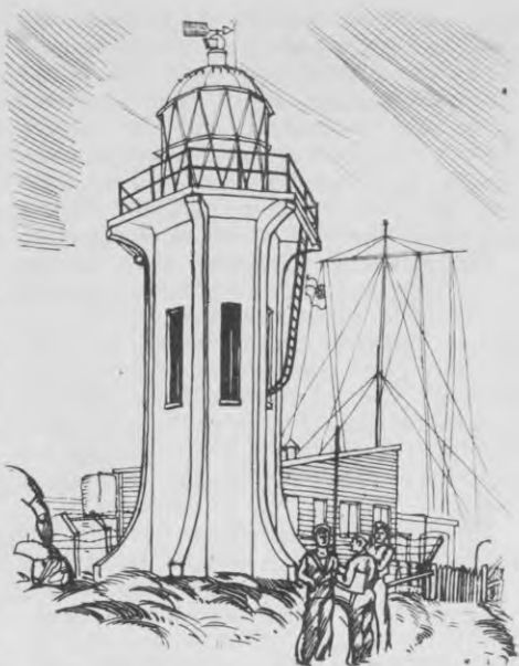
The tower—forty feet of reinforced concrete.
