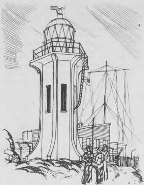
The tower—forty feet of reinforced concrete.
