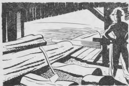
The "fidler" cuts the logs into manoeuvrable lengths.
