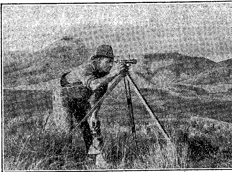
—Christchurch "Times" Photo. ON THE TUSsock-COVERED CANTERBURY HILLS.—A surveyor on the job at Gebbie's Pass, where the new 3YA is in course of erection. One of the masts has now a height approximate to that of the spire of the Christchurch Cathedral—about 220 feet—while the material for the other mast has arrived, and is now being prepared. Each of the towers will weigh 38 tons when completed.
