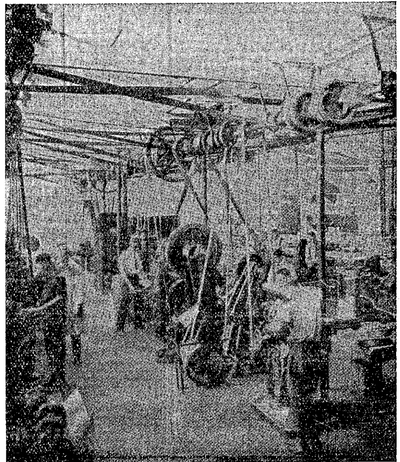
Section of Machine Shop at the A.W.A. Radio Electric Works, Sydney, where all classes of radio transmitting and receiving apparatus are made.
