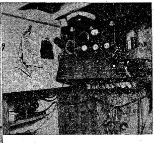
The top of the transmitter in position of the after-bulkhead of the cabin. The dynamo giving the plate supply for the transmitter is seen in the locker at the bottom left. The receiver is below it.
