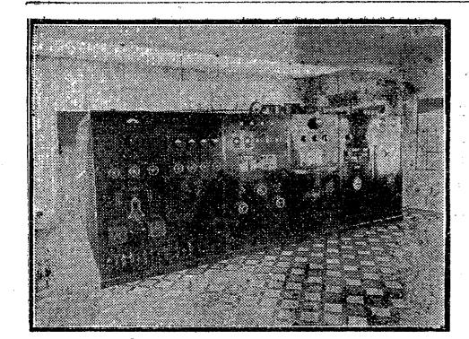
On the left is the 5000-watt transmitter at 2YA. The power is rated on the input to the aerial, making it one of the most powerful transmitting plants in the British Empire.
