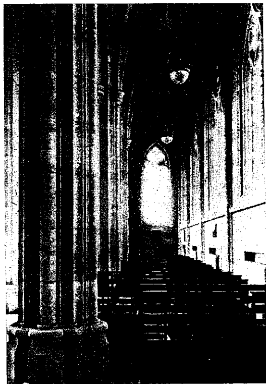
The North Aisle looking "West." Note the base mouldings of the piers, and the caps of the vaulting shafts.
