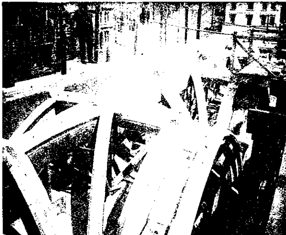
Fig. 5 -Vaulting Ribs of Aisle, Dunedin Cathedral.
