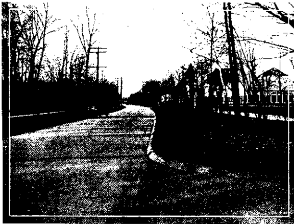
Fig. 27—Sheridan Road, Highland Park, Lake Co., Ill. (Built 1914.) Curbs are built monolithic with Pavement
