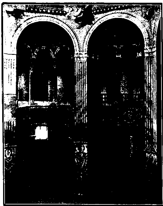
San Vitale from the gallery, showing semi-circular Archings, and semi Vaults under Dome
