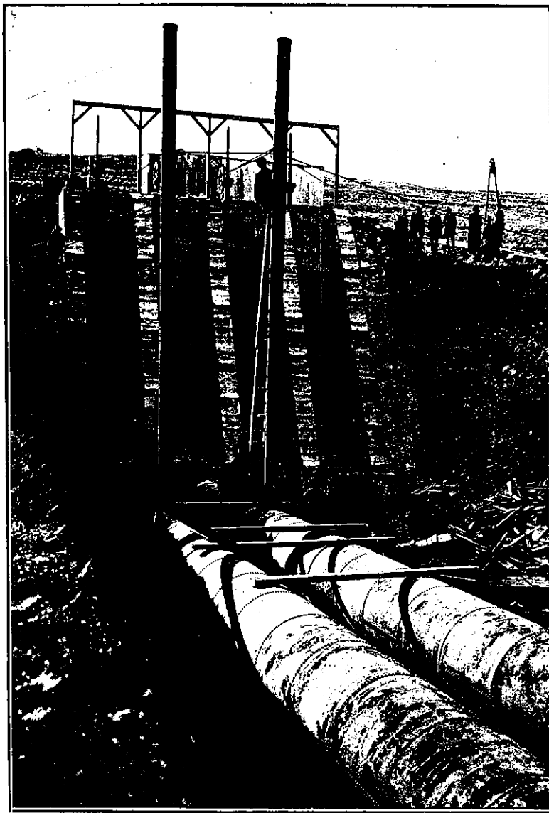
Surge Chamber and Pipe Lines—Erecting the Air Pipes
