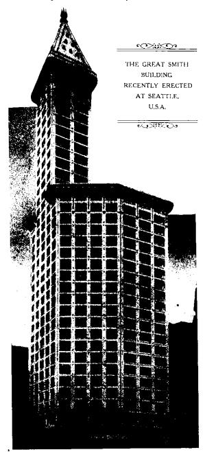
the surface. In building the foundation 4000 barrels of cement and more than 1000 tons of steel were used. On the foundation piles a total weight of 76,560 gross tons will be carried, the steel for the superstructure alone weighing 4732 gross tons.
