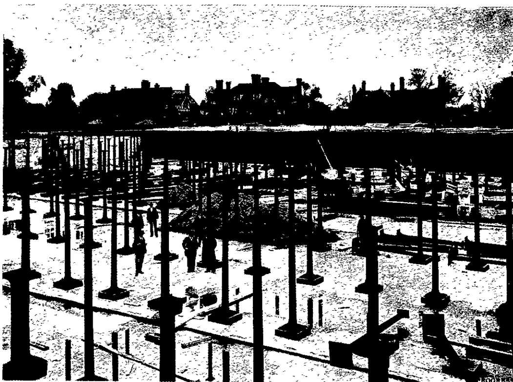
EXPANDED STEEL CONSTRUCTION SHOWING STEELWORK READY TO RECEIVE COVER OF EXPANDED STEEL AND CONCRETE
