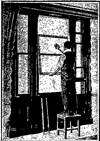
TOP SASH, SWINGING FOR CLEANING.
