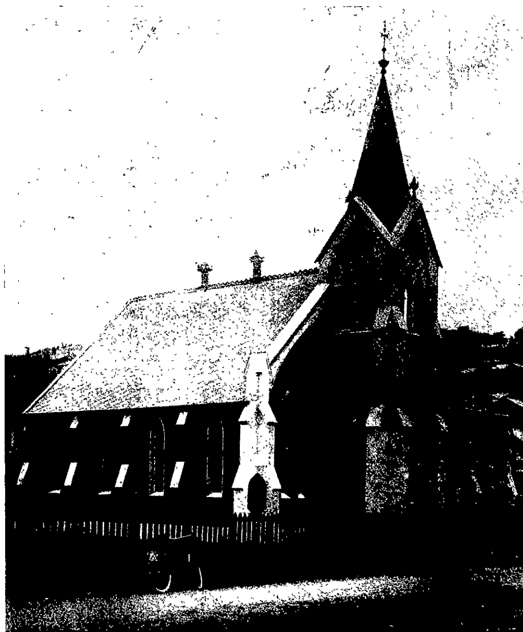
WISLEY CHURCH, GLENAYON, N. F. VALLEY, DUNEDIN. COVERED WITH "FIBRO CEMENT" ASBESTOS SLATES.
