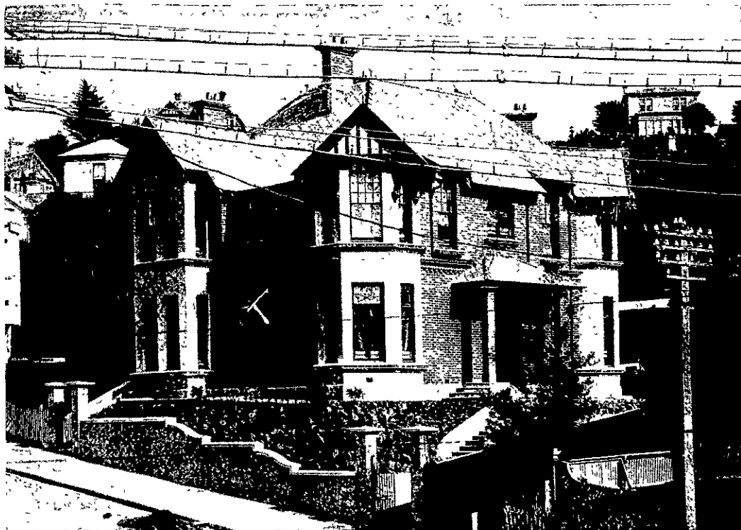
RESIDENCE OF DR BURT, LOWER LONDON STREET, DUNEDIN. COVERED WITH "FIBRO CEMENT" ASBESTOS SLATES. [J. A. Salmond, Architect.]
