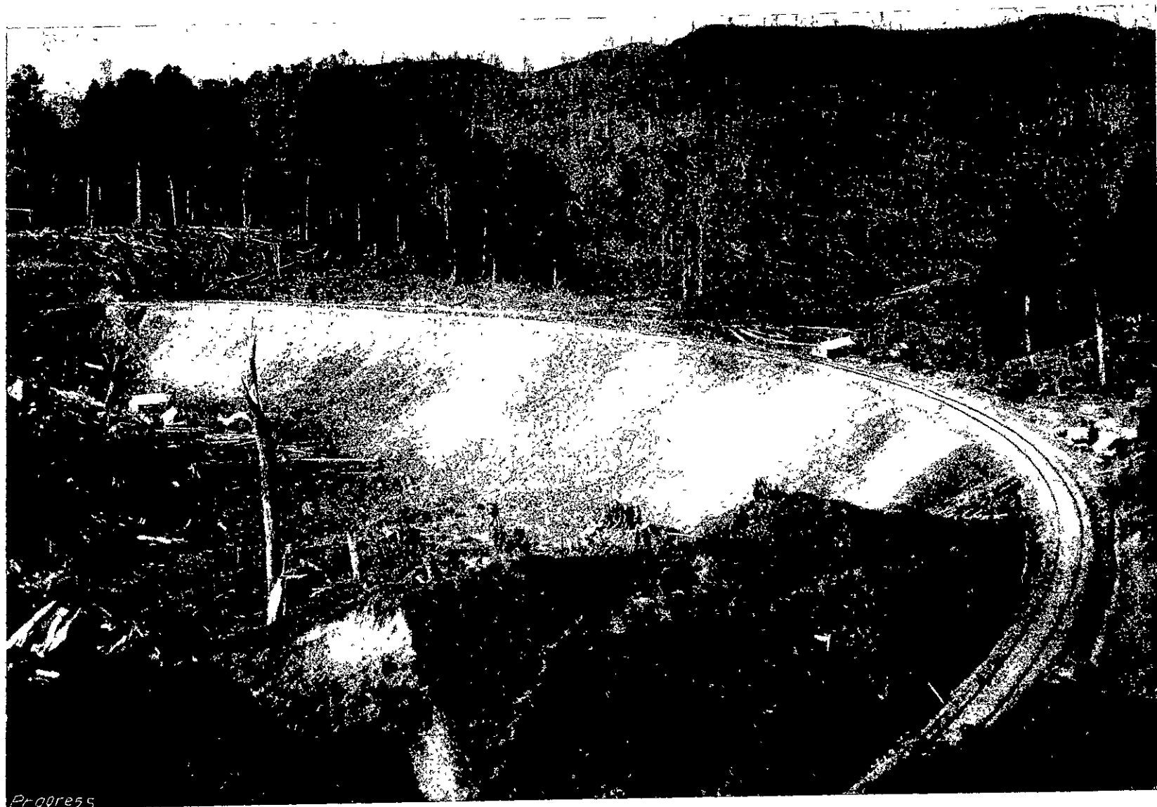
EMBANKMENT, about 2 miles north of Taihape, 63 ft. high; contents, 100,000 cubic yards.
