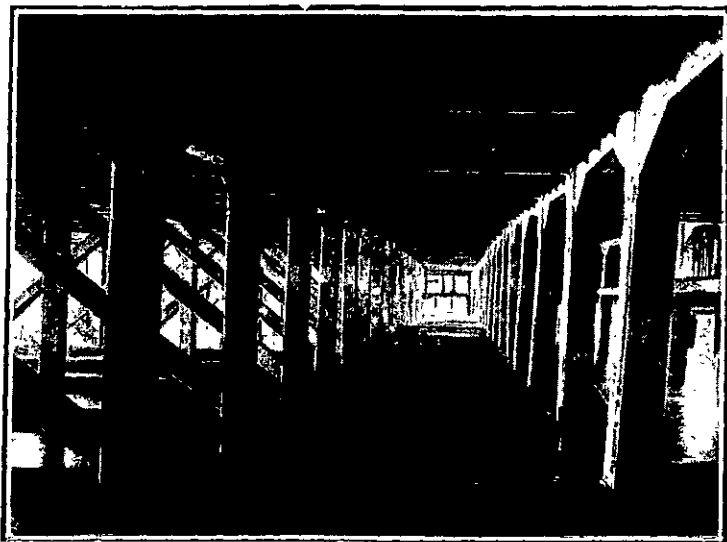
FERRO-CONCRETE WHARF CONSTRUCTION, AUCKLAND: UNDERNEATH VIEW.
