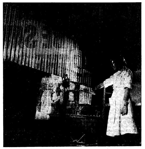
This girl at the Osram Lamp Works of The General Electric Co. Ltd. of England is engaged in the internal coating of fluorescent tubes. A thin cream of fluorescent powder is forced up the tubes by compressed air, and they are then placed on the conveyor (top left) which runs to the drying chamber. The timing of the coating and drying operations is critical because the slightest variation would result
