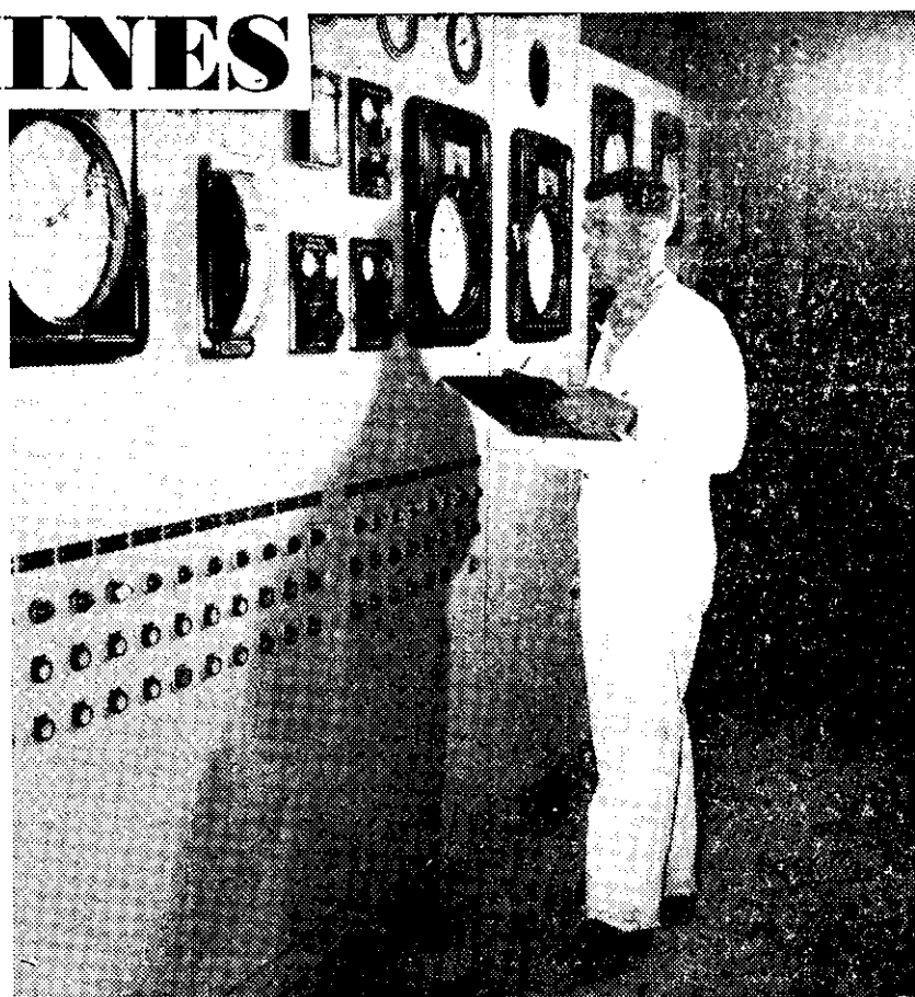
★ "AUTOMATION already exists to some extent in New Zealand"—this photograph, and the one at the foot of the page, show control panels installed at the Kawerau pulp and paper mill.
