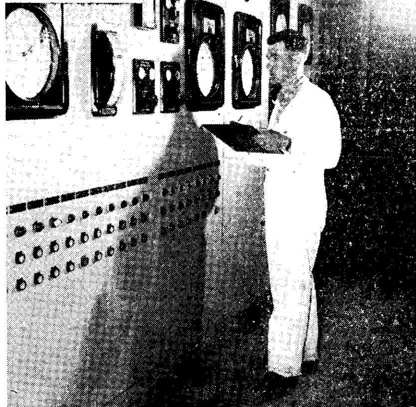
★ "AUTOMATION already exists to some extent in New Zealand"—this photograph, and the one at the foot of the page, show control panels installed at the Kawerau pulp and paper mill.
