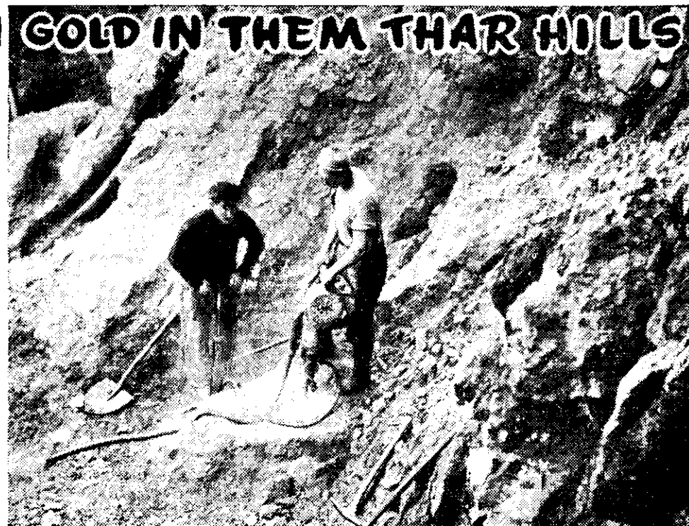
★ MINING mica in the back-country of South Westland. Petrol-driven drilling equipment is shown above and at the foot of the page miners are seen clearing away snow at the 3800-foot level. W. F. Heinz, who took part in this war-time venture, is shown at right ★
