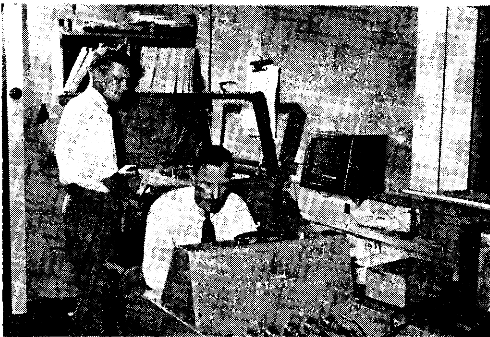
AT TOP: C. G. Wickstead, Sound Director of the National Film Unit, aligning soundtracks on a multiple head moviola. The aligned tracks are then re-recorded on the mixing console, seen in the foreground in the lower photograph
