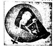
Model "5" "Garrard" Gramophone Units. Model "5" "Garrard" Gramophone Units, consisting of an Electric Gramophone Motor, Constant Speed Rim Drive with a magnetic Pick-up attached. Operates from ordinary light socket or hotpoint. By using one of these units you can play your own records through your ordio set. We've just received them at the new EXCHANGE RATE.
