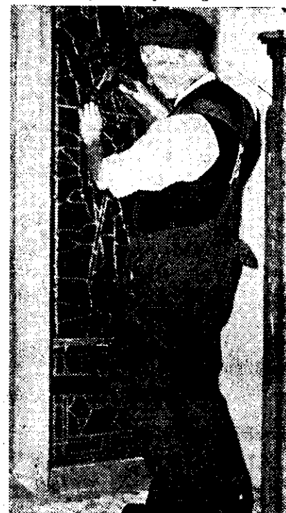
LAST PHASE: A workman fits the top section of a window in a church. Windows must be designed to prevent sagging under the heavy weight of glass and lead
