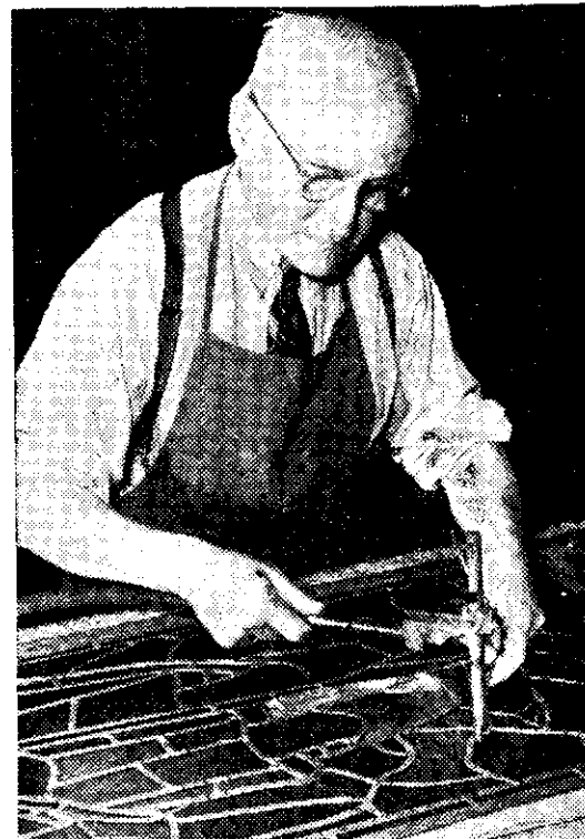
THE PIECES of glass are held together by lead strips, soldered at the joins (as seen above)
