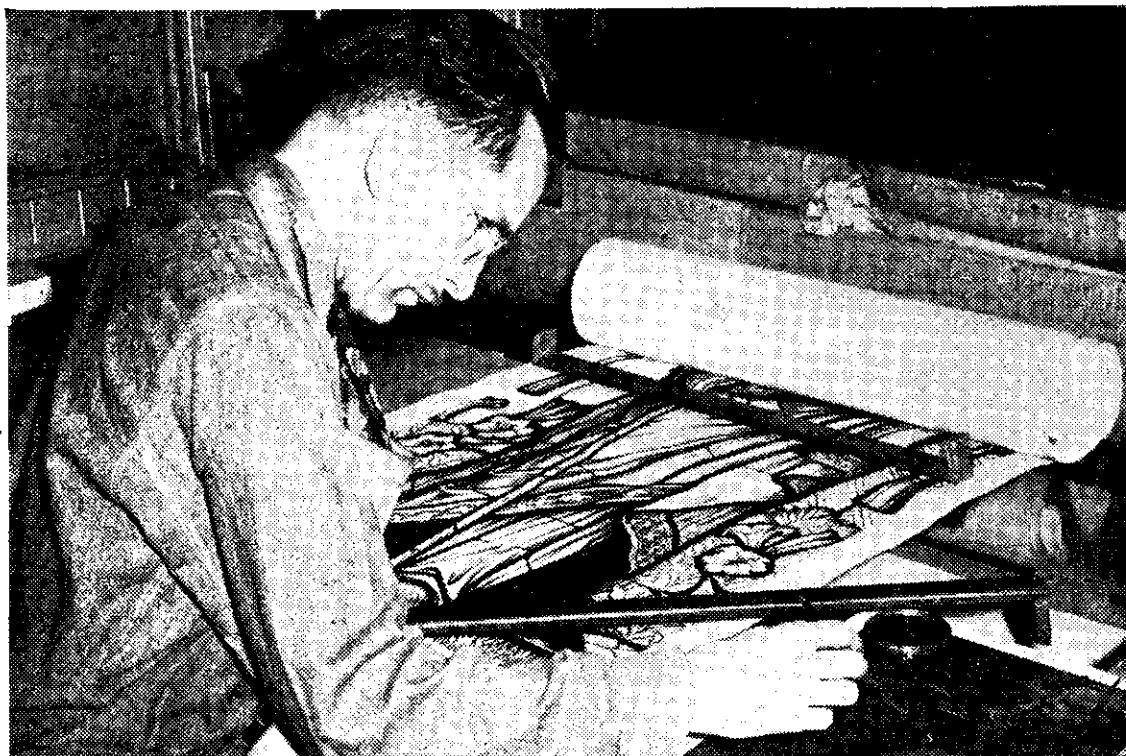
TO PAINT folds in drapery, flowers, and other details, the glass to be used is placed directly over the cartoon
