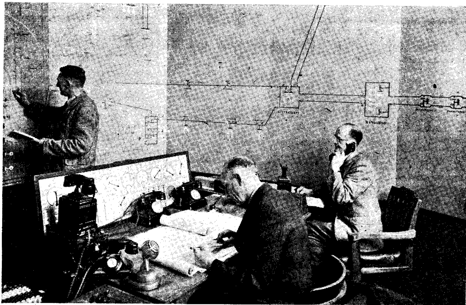
OPERATION BLACKOUT: A scene in the electricity load despatch office at Hamilton from which the distribution of electric power throughout the North Island is controlled (see page 14)
