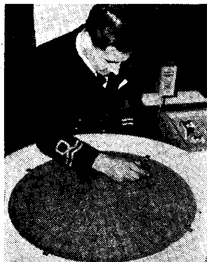
The Radar "Skyboard" used by the Navy to plot the positions of aircraft.
