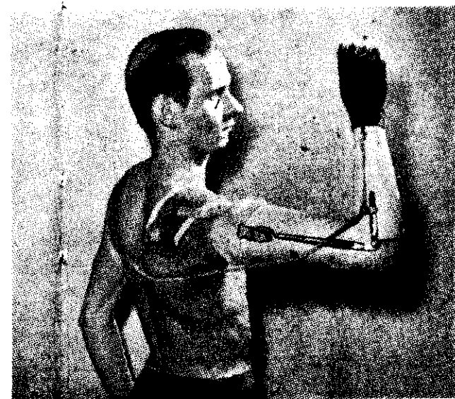
Artificial arm is made of plastic and metal to lessen weight. To bend arm at elbow, the soldier contracts muscles of his back, which pull on a leather thong attached to his wrist.
