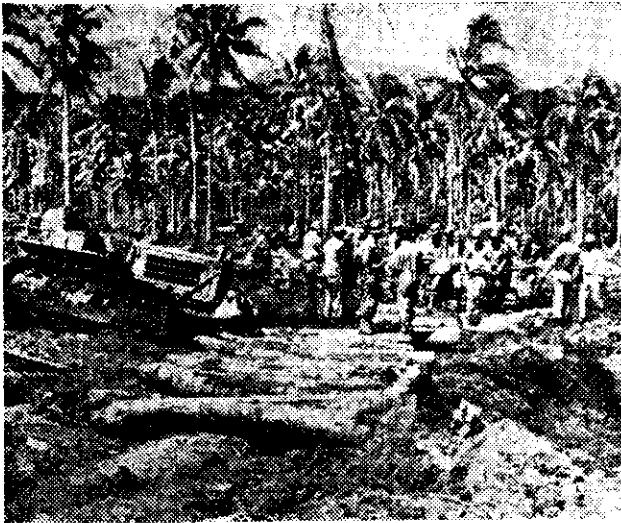
IN JUNGLE MUD on Rendova Island in the Solomons a palm grove is cut down to make logs for a corduroy road.
