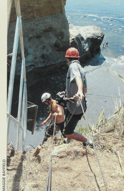
Abseiling to construct the fence. The protected area ends at the cliff face with a projecting fence to exclude pests which kill the burrow-nesting birds.
