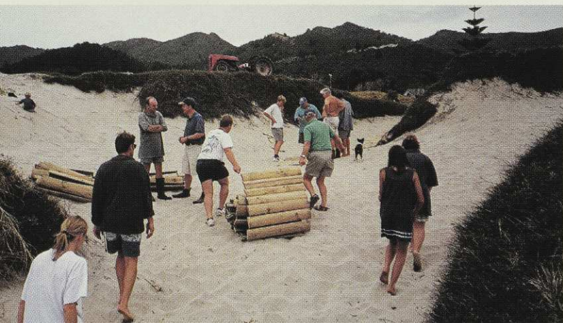
Installing a boardwalk to protect sand dunes at Medlands Beach, at Great Barrier Island.
