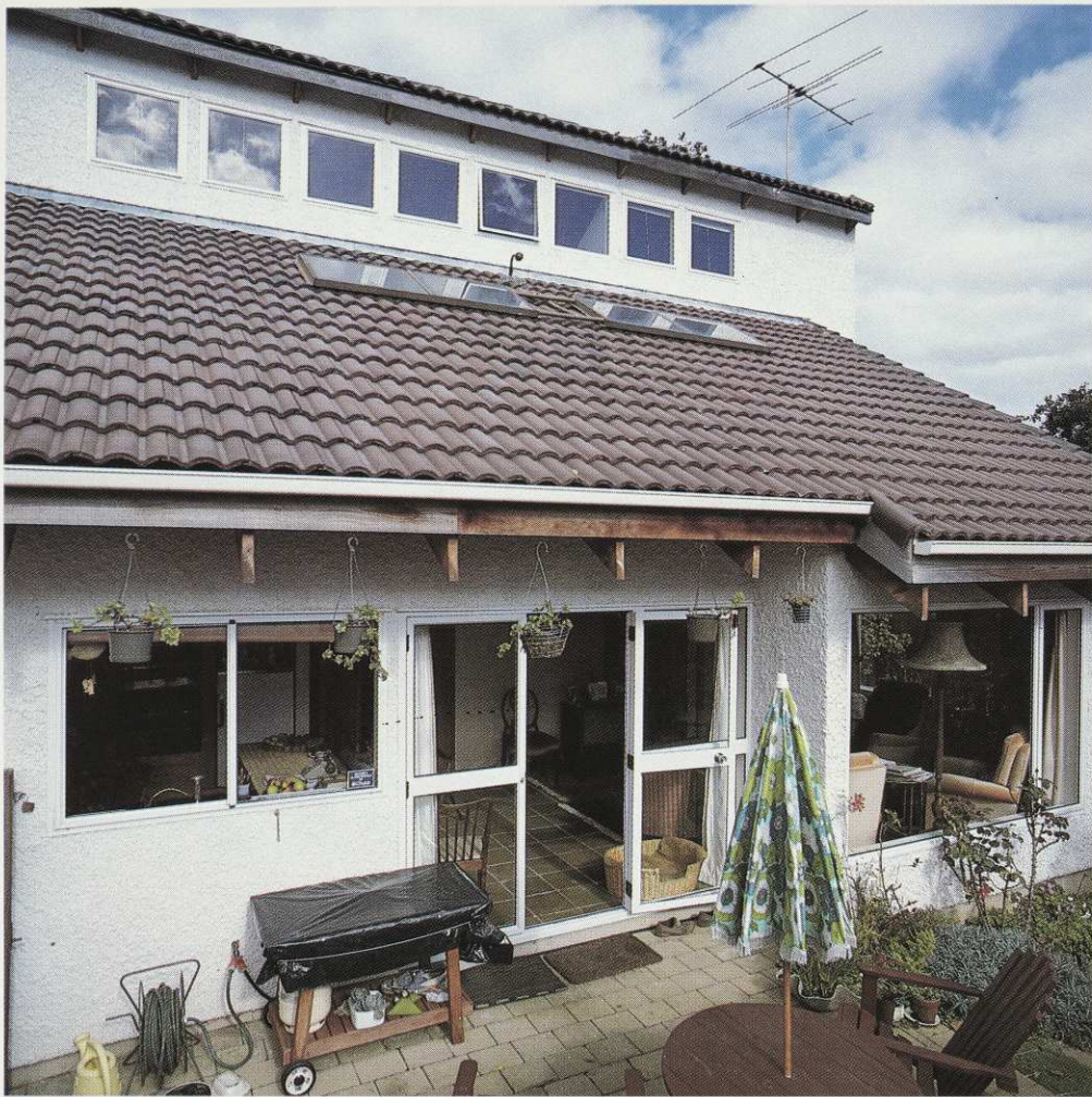
A home built for the sun, with solar panels and direct gain. It has been estimated that such simple efficiency measures in New Zealand homes would free up energy equivalent to 12 power stations the size of the scrapped Luggate dam. Photo: Energy Management Group
