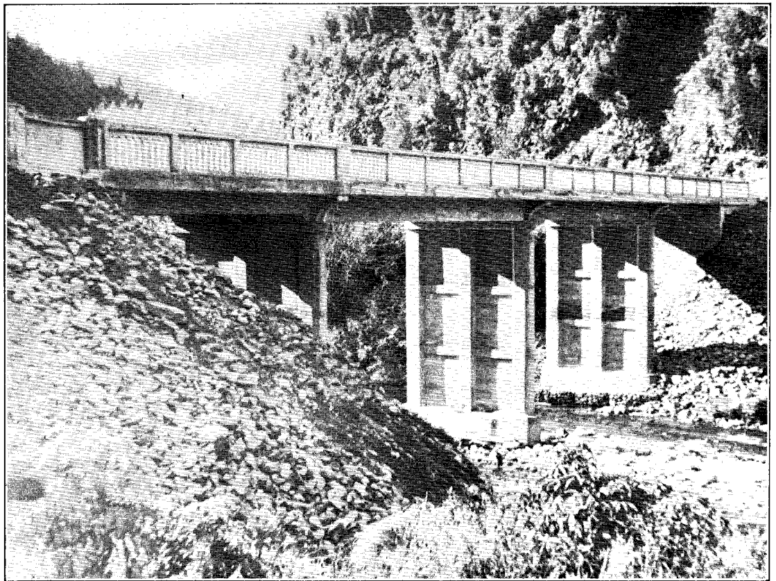
OHIWA-ITI RIVER BRIDGE, BULLER GORGE. TWO 30 FT. AND TWO 45 FT. SPANS, 20 FT. ROADWAY. NELSON-WESTPORT STATE HIGHWAY.
