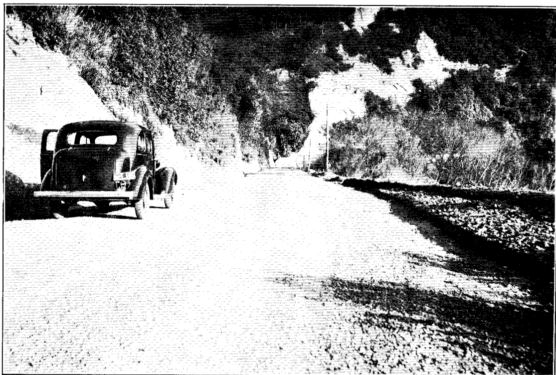
SECTION OF BITUMEN-SEALING ON RECONSTRUCTED LENGTH. NATIONAL PARK—WANGANUI STATE HIGHWAY.
