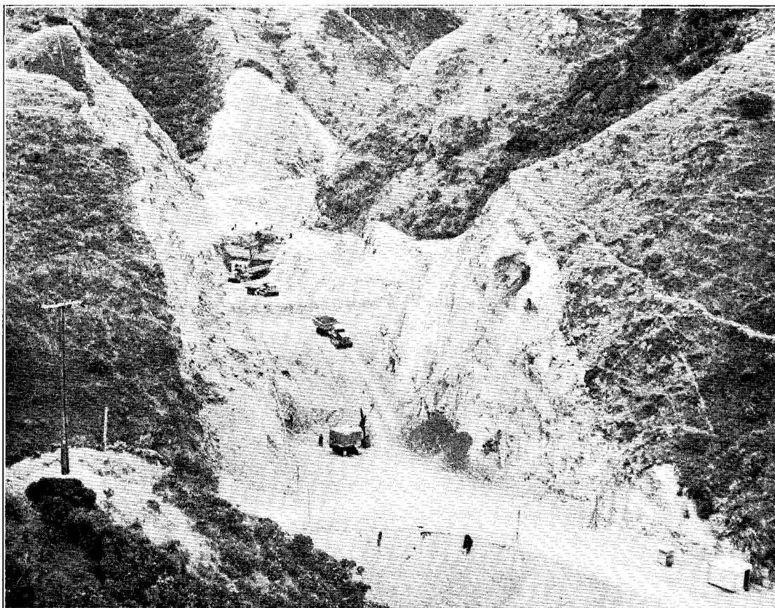
VIEW OF THE MAIN CUTTING LOOKING TOWARDS JOHNSONVILLE. FINAL ALIGNMENT OF THIS SECTION IS ON A 15-CHAIN-RADIUS CURVE. BATTERS ON LEFT WILL BE 145 FT. AND 160 FT.
