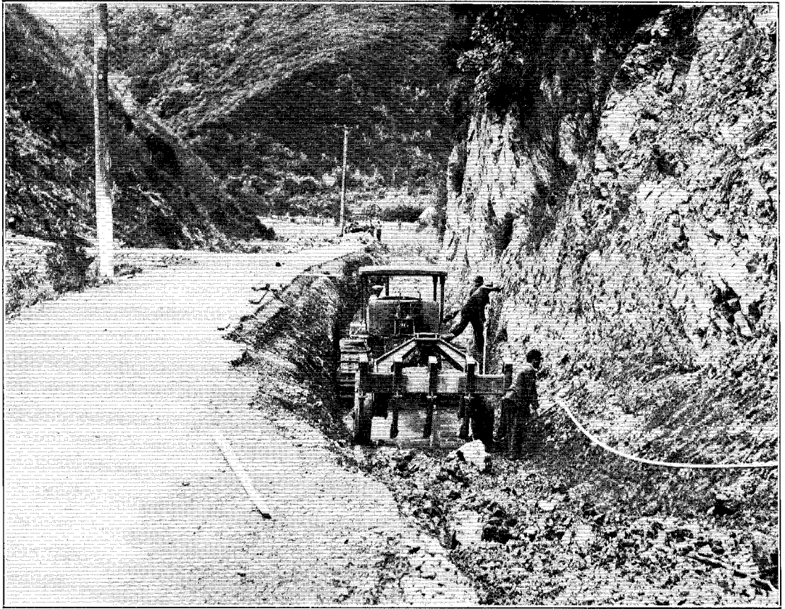
CATERPILLAR TRACTOR OPERATING ROCK ROOTER IN TRENCH FOR CREEK-DIVERSION.
