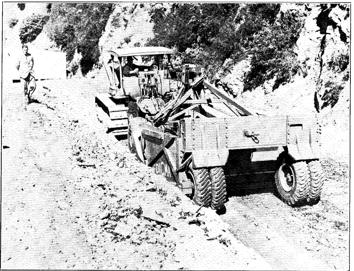
CATERPILLAR TRACTOR OPERATING CARRYALL SCRAPER ON EXCAVATION OF TRENCH FOR BASE OF TWIN 6-FT.-DIAMETER CONCRETE PIPES.
