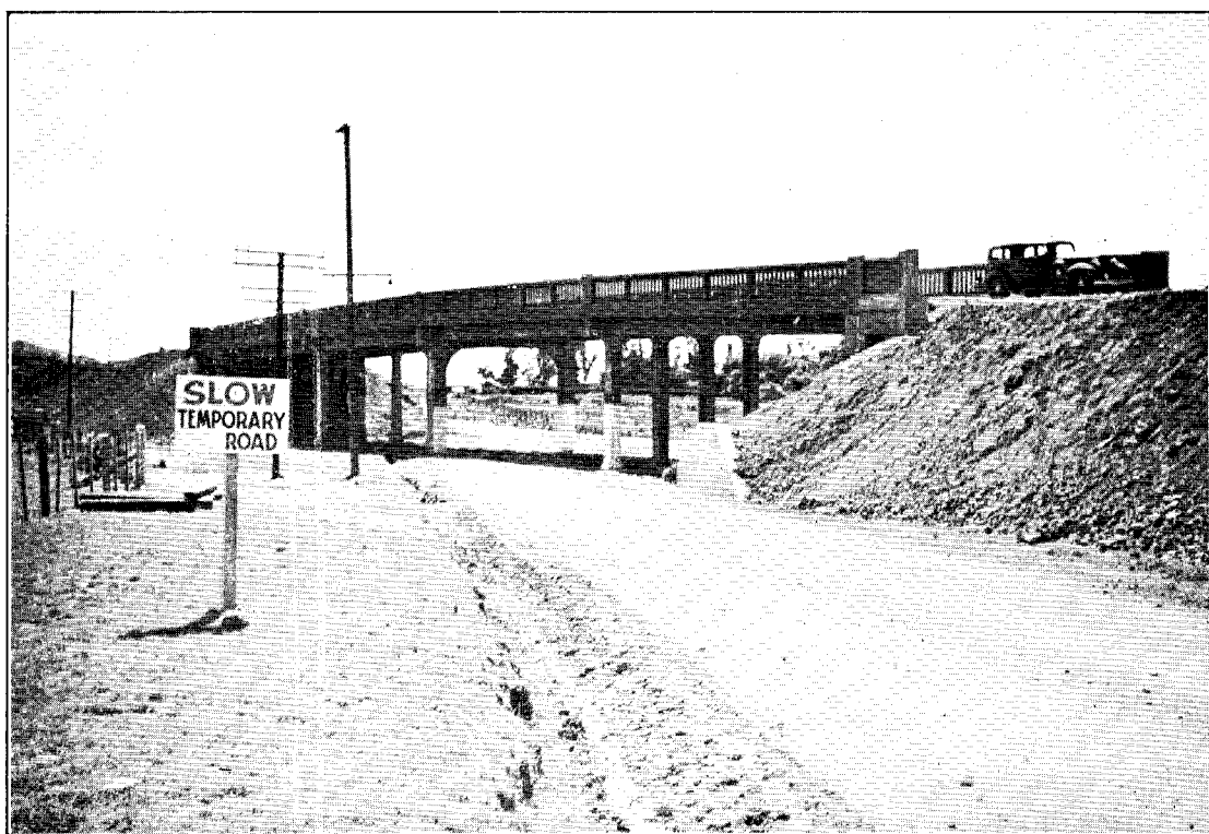
LEVEL-CROSSING ELIMINATION, OVERBRIDGE, 10 M. 49 CH. RAILWAY FORMATION IN USE AS TEMPORARY ROAD.
