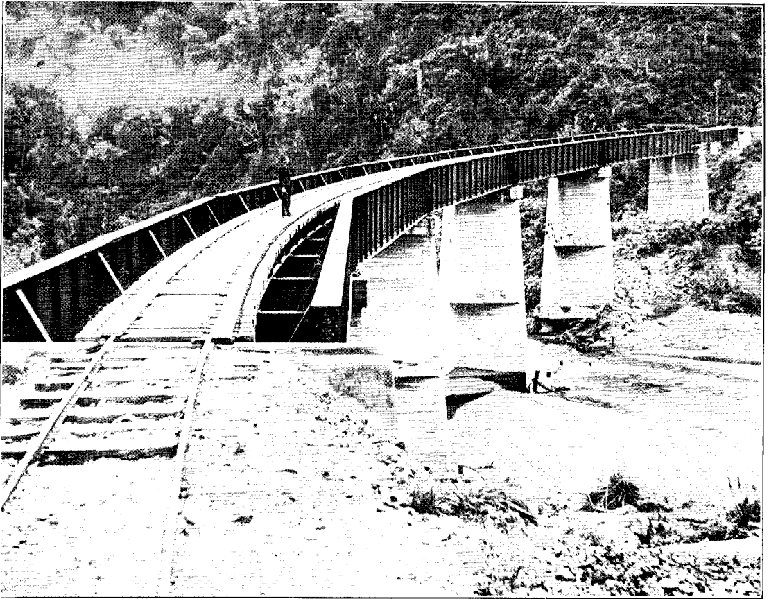
CASCADE CREEK BRIDGE. FIVE 80 FT. AND ONE 40 FT. PLATE-GIRDER SPANS ON 7\frac{1}{2} CHAINS RADIUS CURVE.
