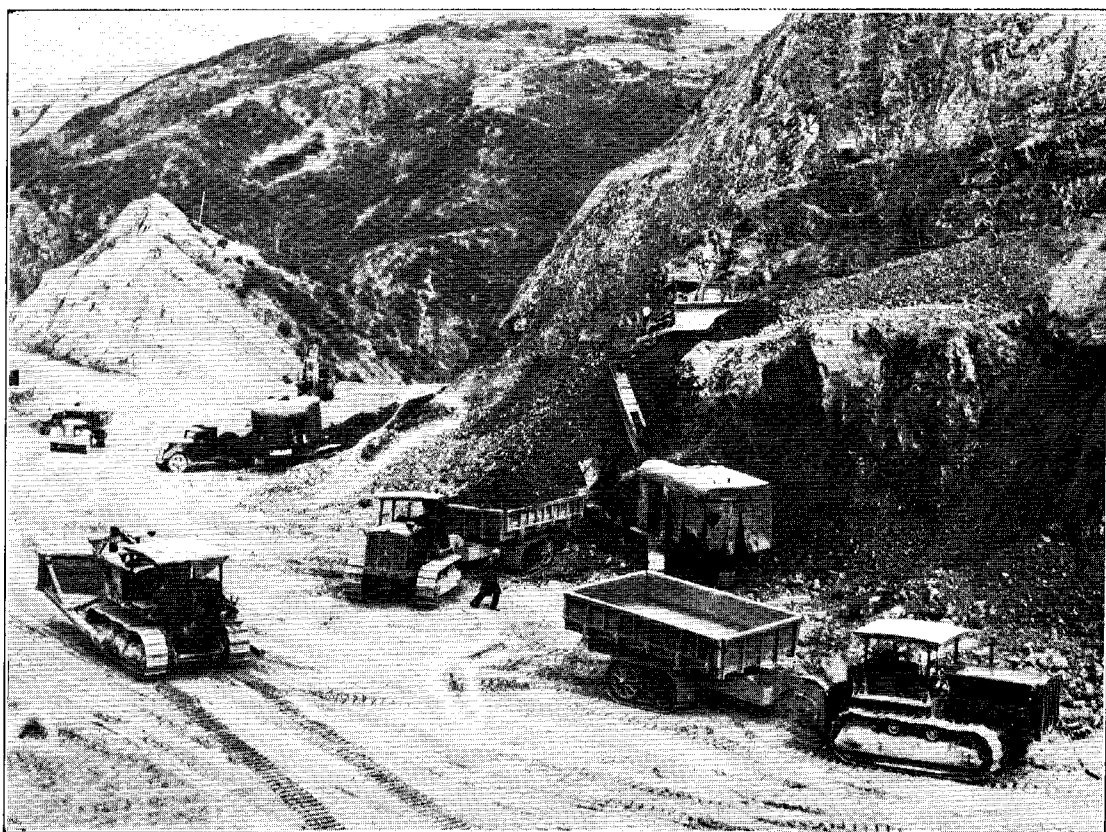
EXCAVATING AND HAULING EQUIPMENT IN OPERATION. NGAHAURANGA GORGE ROAD. WELLINGTON-TAWA FLAT MAIN HIGHWAY.
