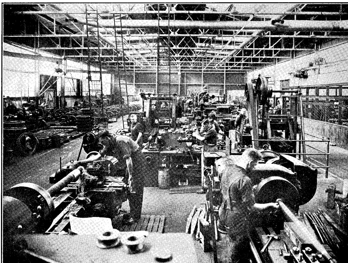
OTAHUHU CAR AND WAGON WORKSHOPS : MACHINE SHOP.
