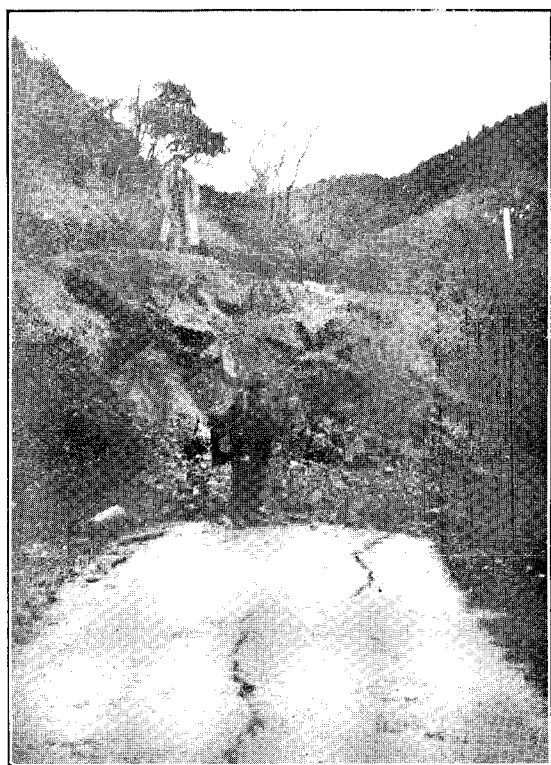
3. "UPTHROW" OF ROAD (13 FT. 5 IN.) WHERE CROSSED BY EARTHQUAKE FAULT-LINE NEAR WHITE'S CREEK, BULLER GORGE.
