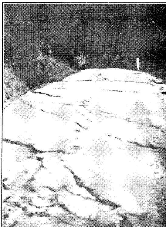
4. FISSURES AND PRESSURE-RIDGES ON BULLER GORGE ROUTE.
