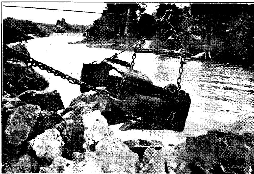
Drag-line Bucket in Rock, No. 1 Bar.
