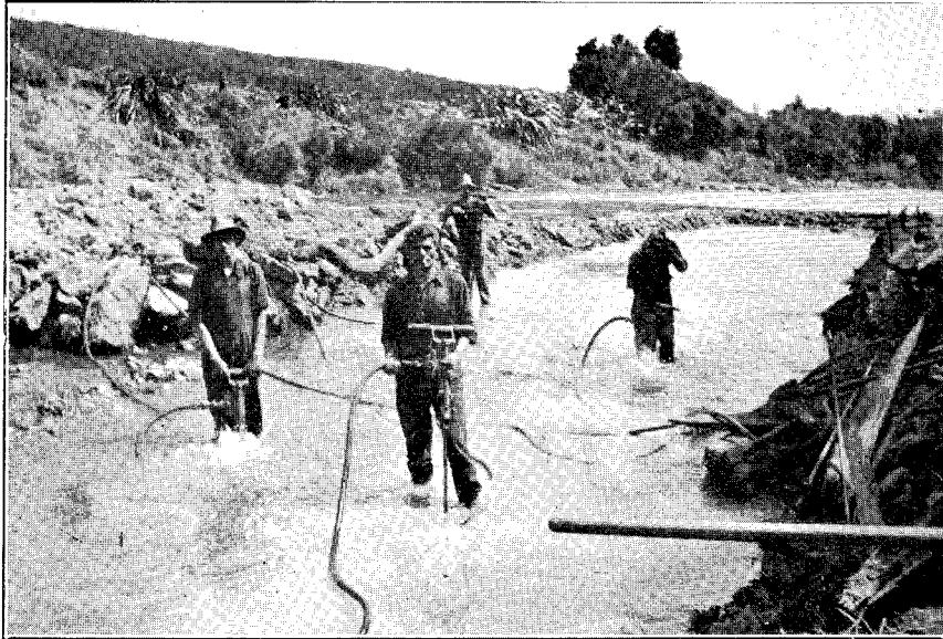
Rock-drilling on No. 2 Bar, Wairua River.
