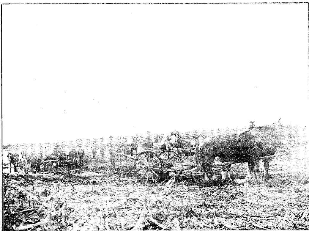
WHEEL SCOOPS AT WORK ON OMERU OUTFALL.
