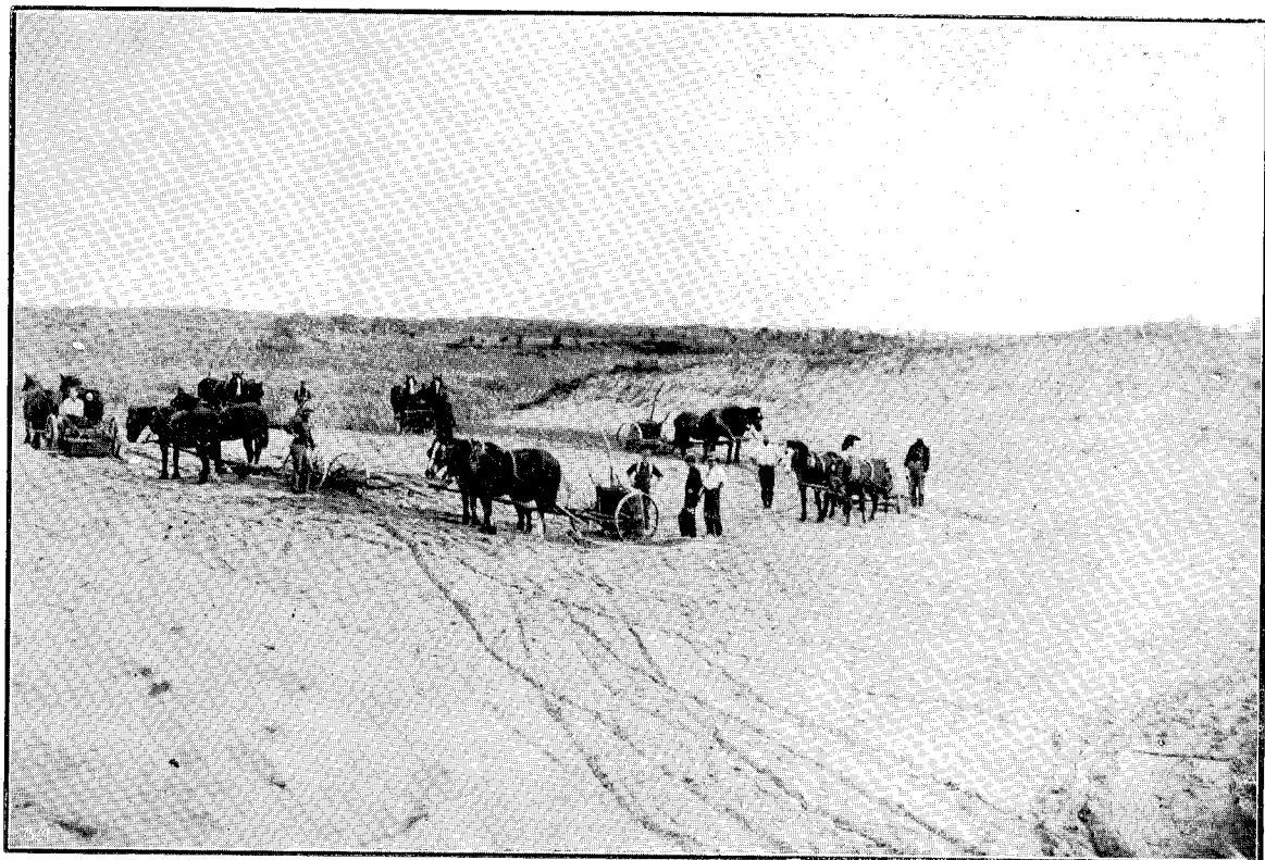
RANGITAHI RIVER DIVERSION.—SCOOP TEAMS EXCAVATING SANDHILLS.
