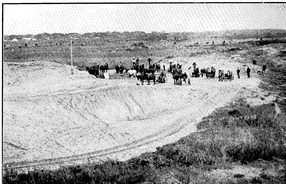
RANGITAKI RIVER DIVERSION.—SCOOP TEAMS AT WORK ON EXCAVATION OF SANDHILLS.
