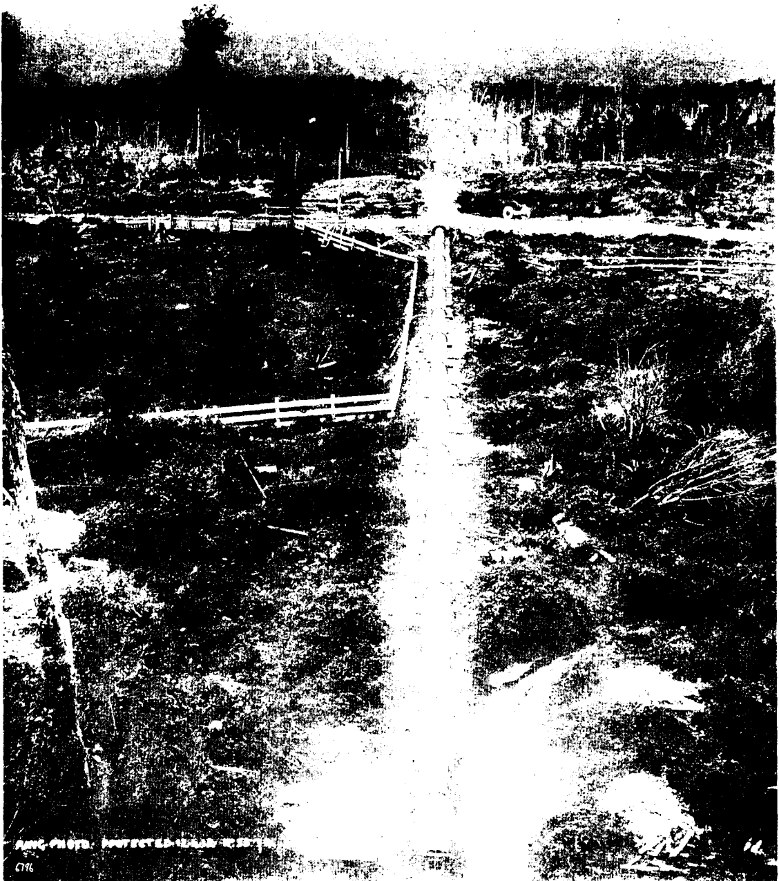
KUMAYA GOVERNMENT MINING WATER P.W.C. EXTENSION. INVERTED SIPHON OF 30 INCH BORE, 2 MILES 1 CHAIN IN LENGTH, CROSSING THE VALLEY OF THE RIVER TARAMALAI, WESTLAND.
