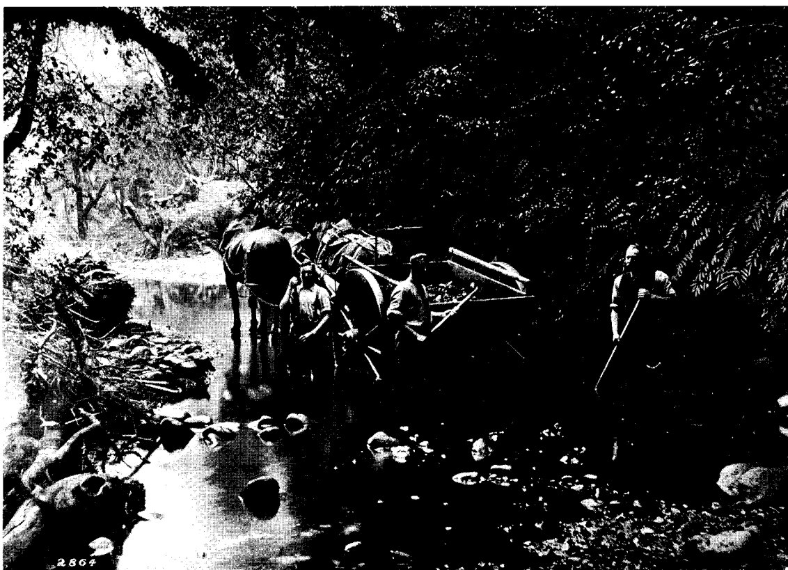
GETTING SHINGLE FOR CONCRETE-WORK, NORTH ISLAND MAIN TRUNK RAILWAY.
