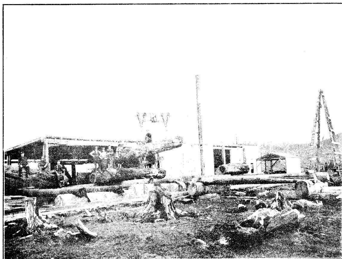
[No. 18.] Overhead Apparatus for Hauling Logs, Nipawin, Okeechewee Bay
