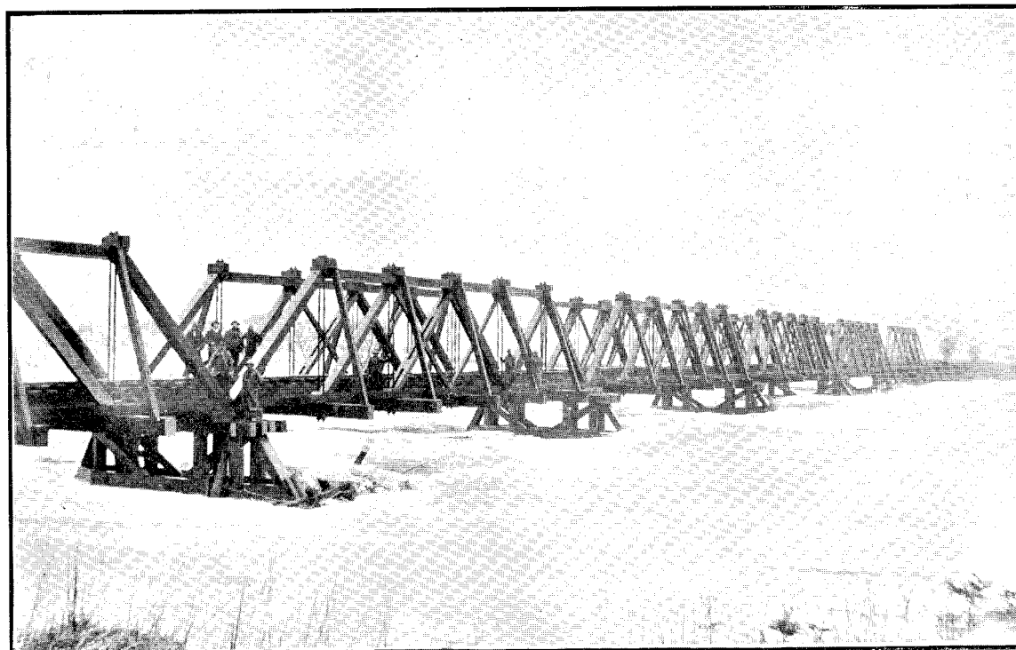
GISBORNE—ROTORUA RAILWAY.—BRIDGE OVER WAIPAQA RIVER AT KATTERATAHI DURING FLOOD OF 16TH AND 17TH JULY, 1906, AFTER FLOOD HAD SUBSIDED 4 FT.
