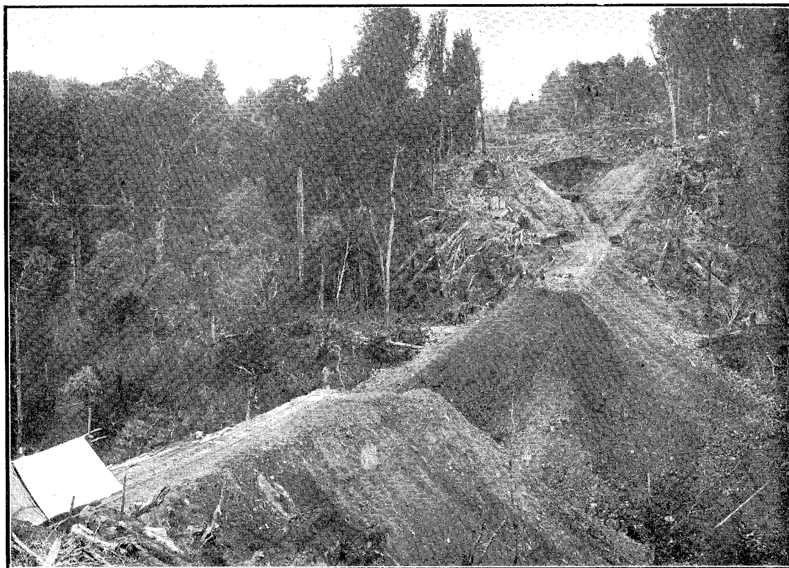
NORTH ISLAND MAIN TRUNK RAILWAY.—BANK OVER WAIKAKARIKI WATER-TUNNEL, AT 115 M. 48 CH. (ABOUT 70 FT. HIGH).
