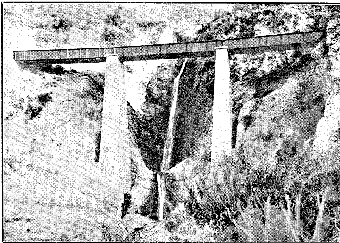
NEW ZEALAND MIDLAND RAILWAY. — BRIDGE OVER ROCKY CREEK, AT 11 M. 61 CH. FROM SPRINGFIELD. (THREE SPANS OF 44 FT., ON CONCRETE PIERS 66 FT. HIGH.)
