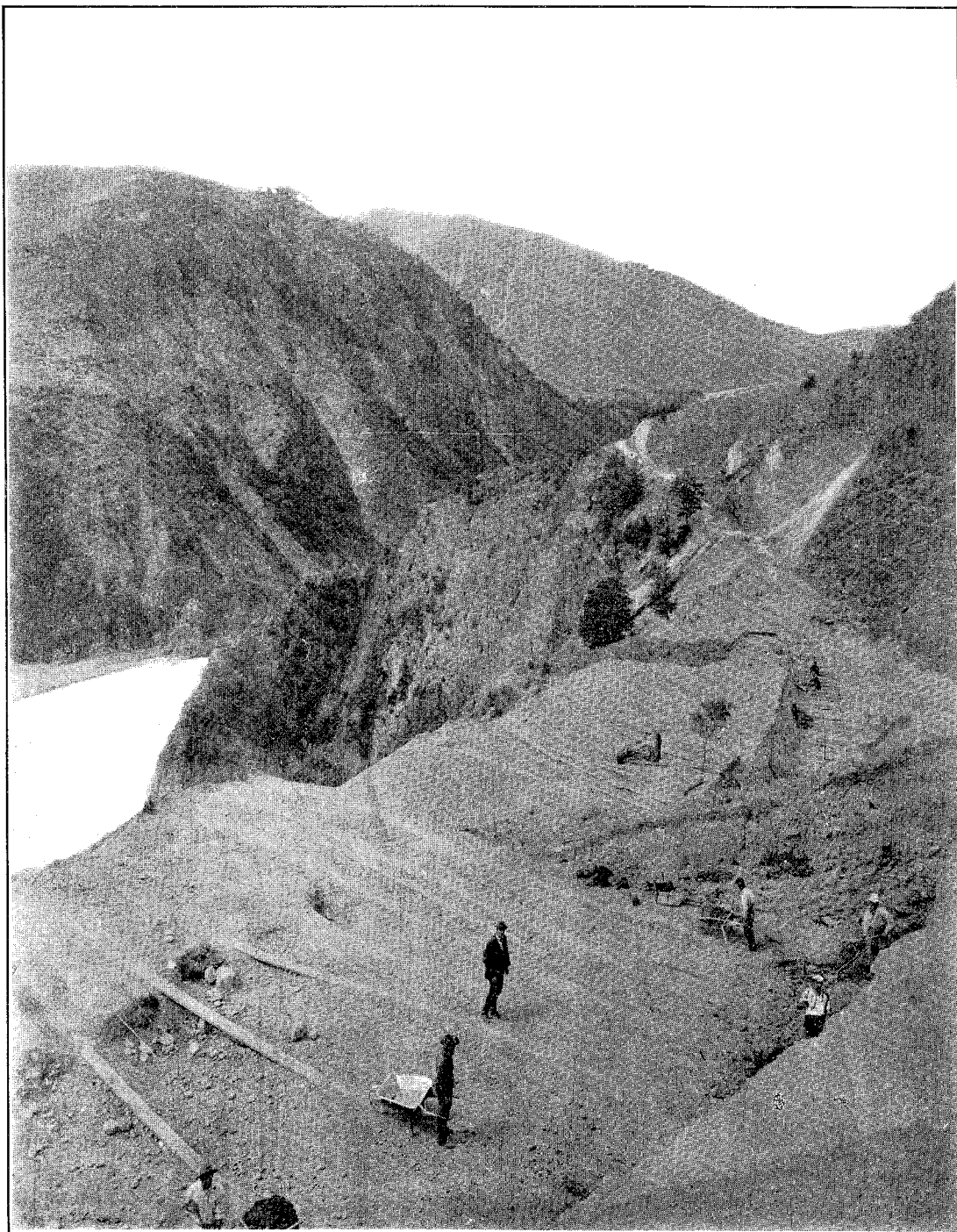
Midland Railway, Mount Torlesse Section : 60 ft. cutting, and spoil-bank at 9 miles 66 chains.
