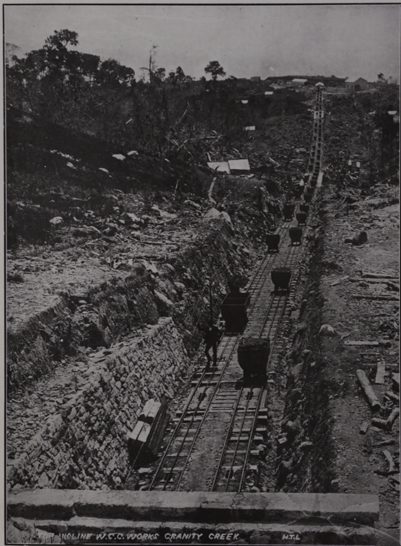
UPPER PART OF WESTPORT COAL COMPANY'S INCLINE, GRANITY TO MILLERTON. Geol. Bull. No. 17.]
