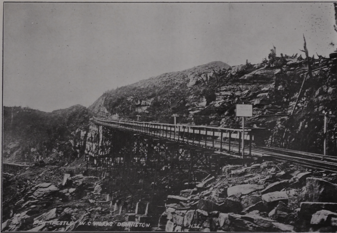
IRON TRESTLE, WESTPORT COAL COMPANY'S HAULAGE ROAD, DENNISTON. THE VIEW SHOWS NEARLY HORIZONTALLY BEDDED COAL-MEASURE ROCKS. THE ROAD TO THE OLD BANBURY MINE IS SEEN ON THE LEFT.
