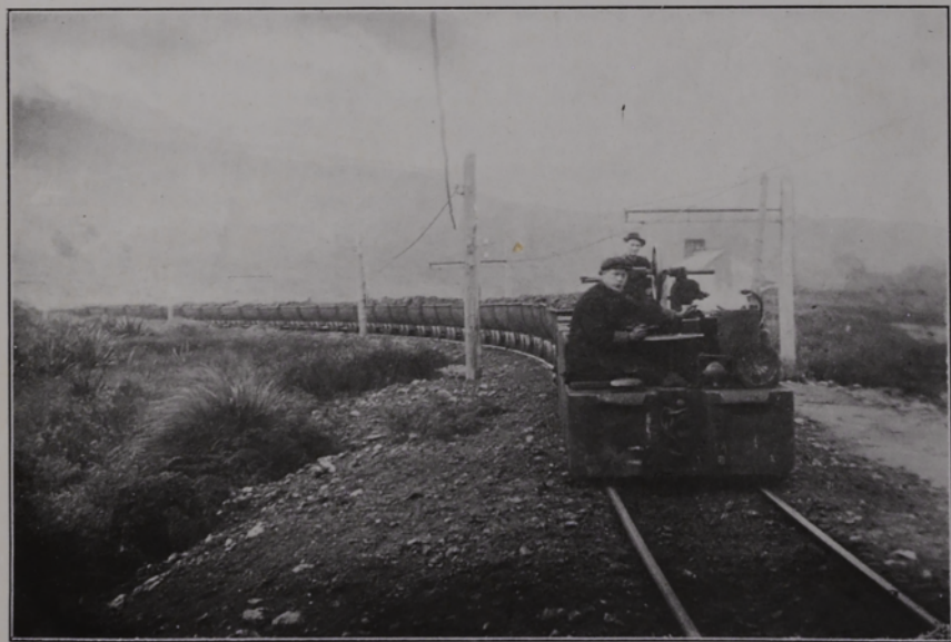
ELECTRIC LOCOMOTIVE BRINGING RACE OF LOADED TUBS FROM WESTPORT-STOCKTON COMPANY'S MINE TO TOP OF INCLINES.
