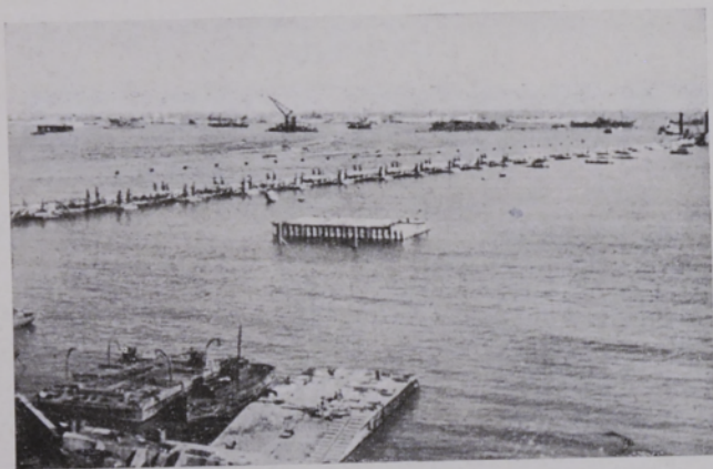
"BIGGER THAN DOVER." Mobile Harbour at Normandy Beach-head. June, 1944.
